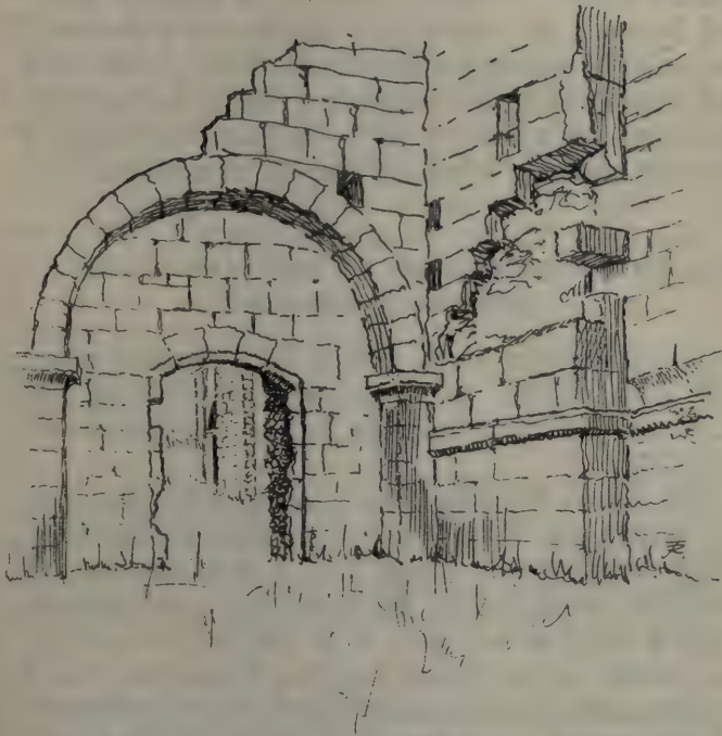
FIG. 62. DOORWAY FROM LOBBY TO TREASURY.
